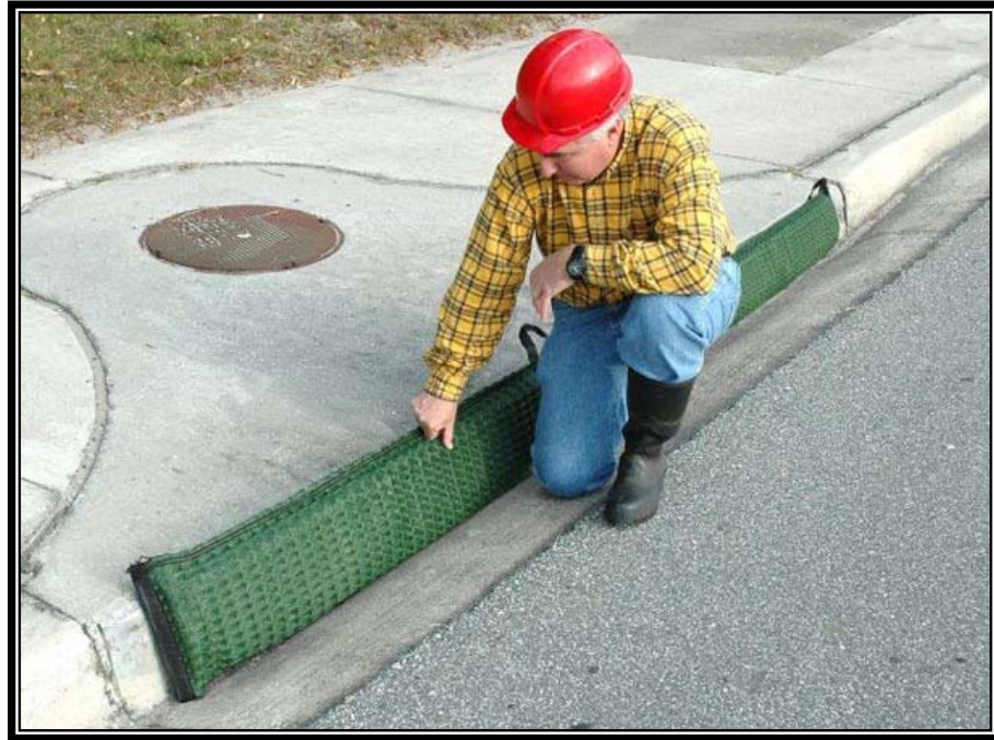
Figure 4.20. Commercially Available Gutter Guard Being Replaced.
