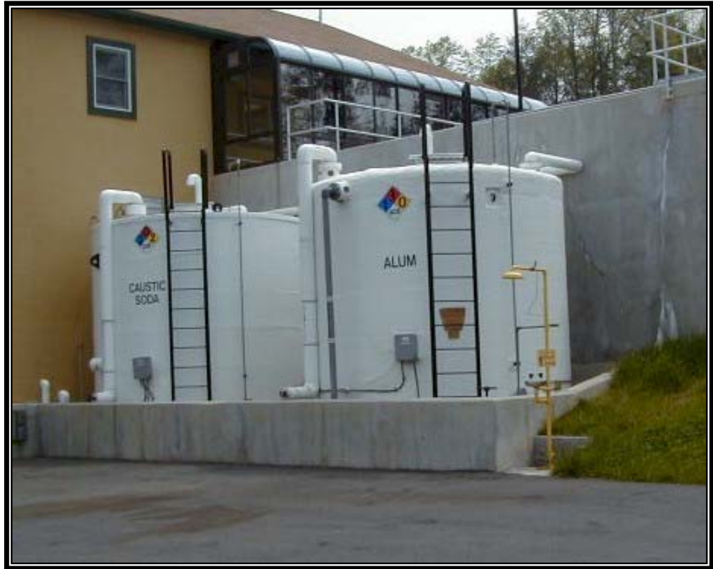
Figure 4.19. Aboveground Storage Tanks with Secondary Containment.
