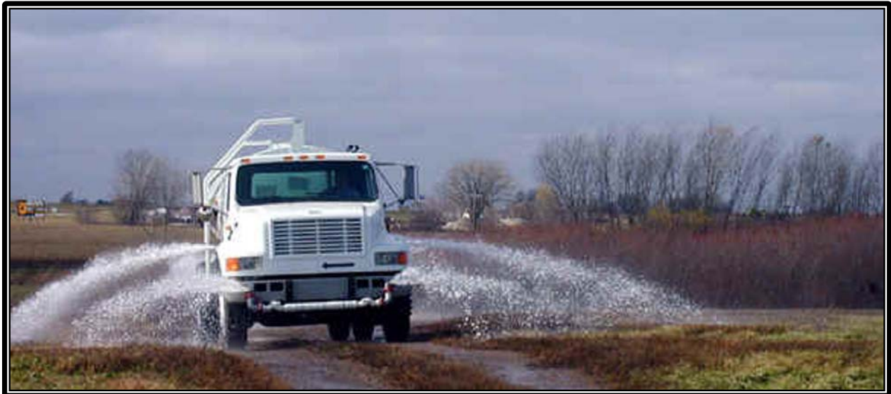
Figure 4.21. Dust Suppression by Water Spray.
