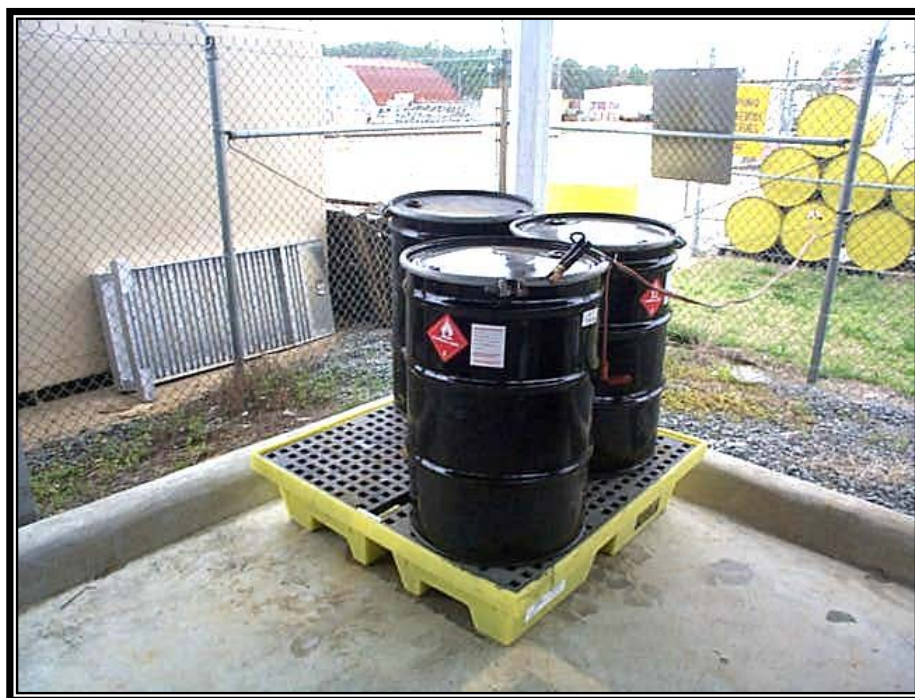
Figure 4.17. Temporary Secondary Containment.
