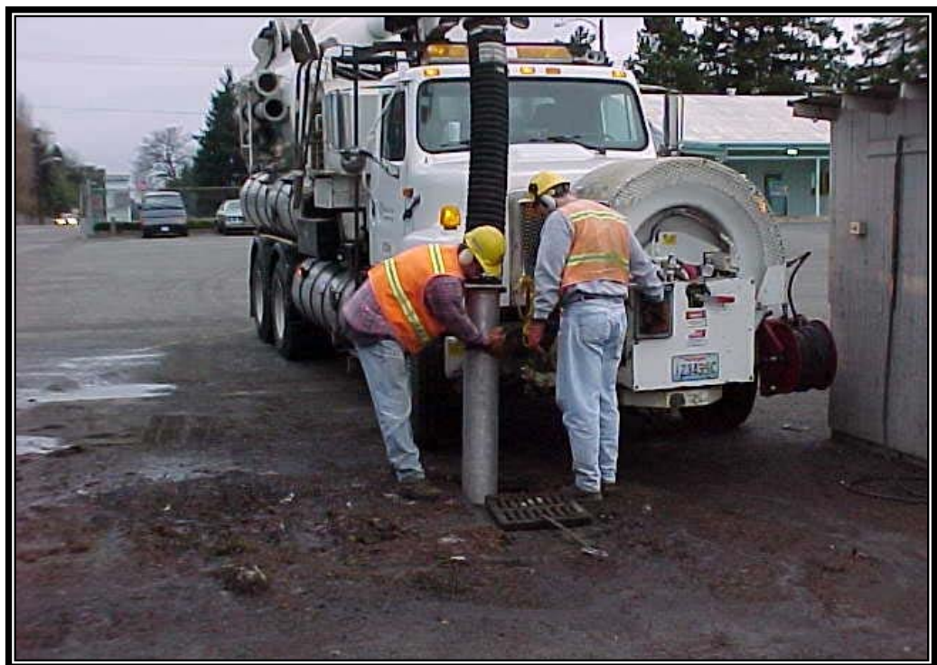
Figure 4.23. Catch Basin Cleaning with a Vacuum Truck.
