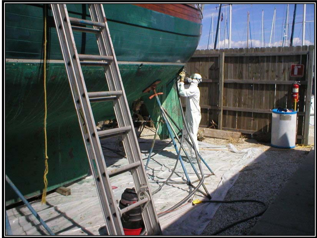
Figure 4.22. Drop Cloth Used During Hull Sanding.
