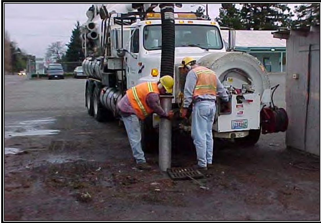
Figure 5.8. Catch Basin Cleaning with a Vacuum Truck.
