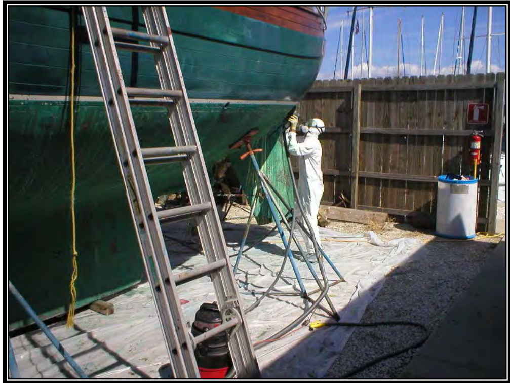
Figure 4.22. Drop Cloth Used During Hull Sanding.
