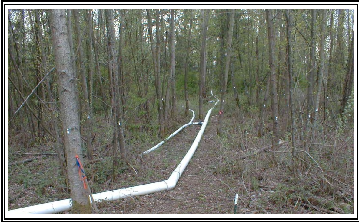
Figure 3.14. Manifold and Branches in a Wooded, Vegetated Spray Field
