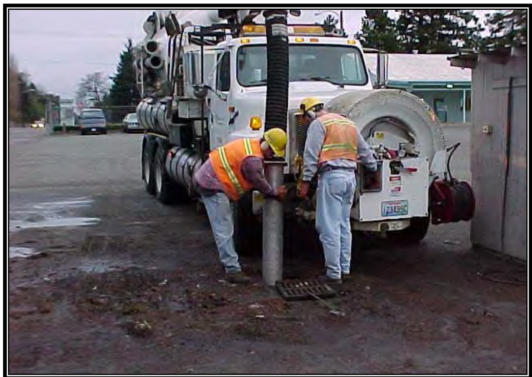
Figure 4.23. Catch Basin Cleaning with a Vacuum Truck.
