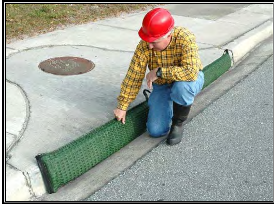
Figure 4.20. Commercially Available Gutter Guard Being Replaced.
