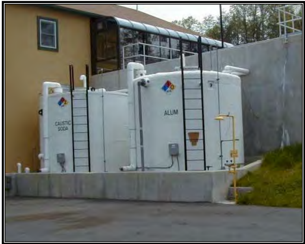
Figure 4.19. Aboveground Storage Tanks with Secondary Containment.
