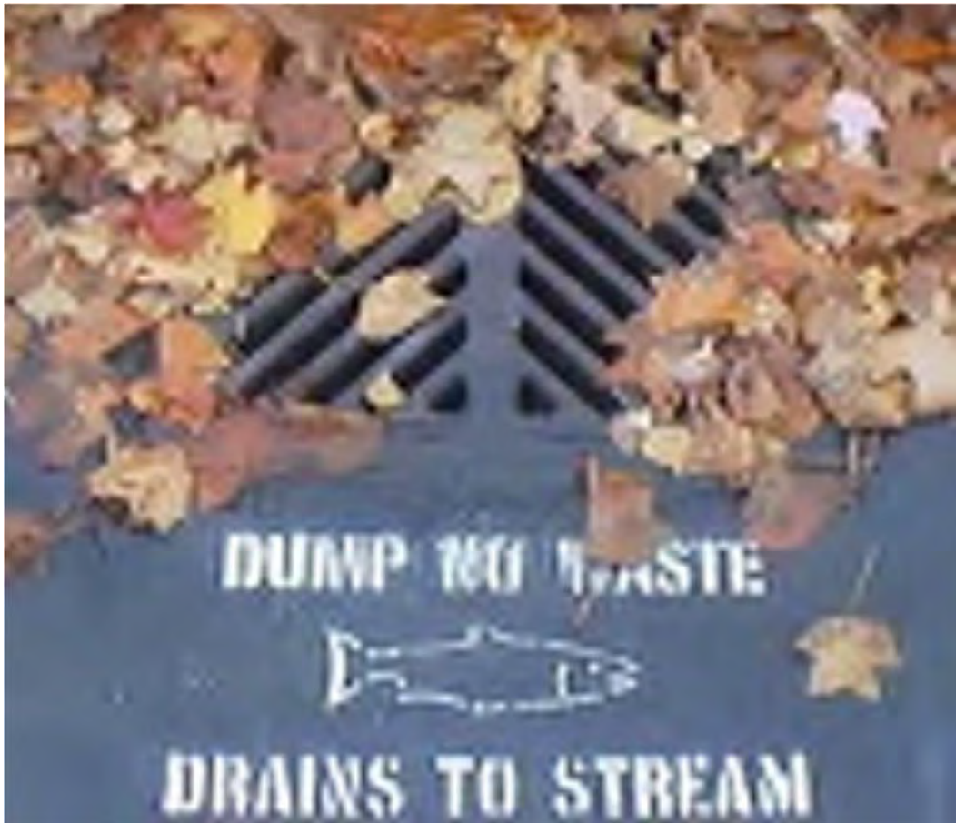
Figure 5.9. “Dump No Waste” Storm Drain Stencil.
