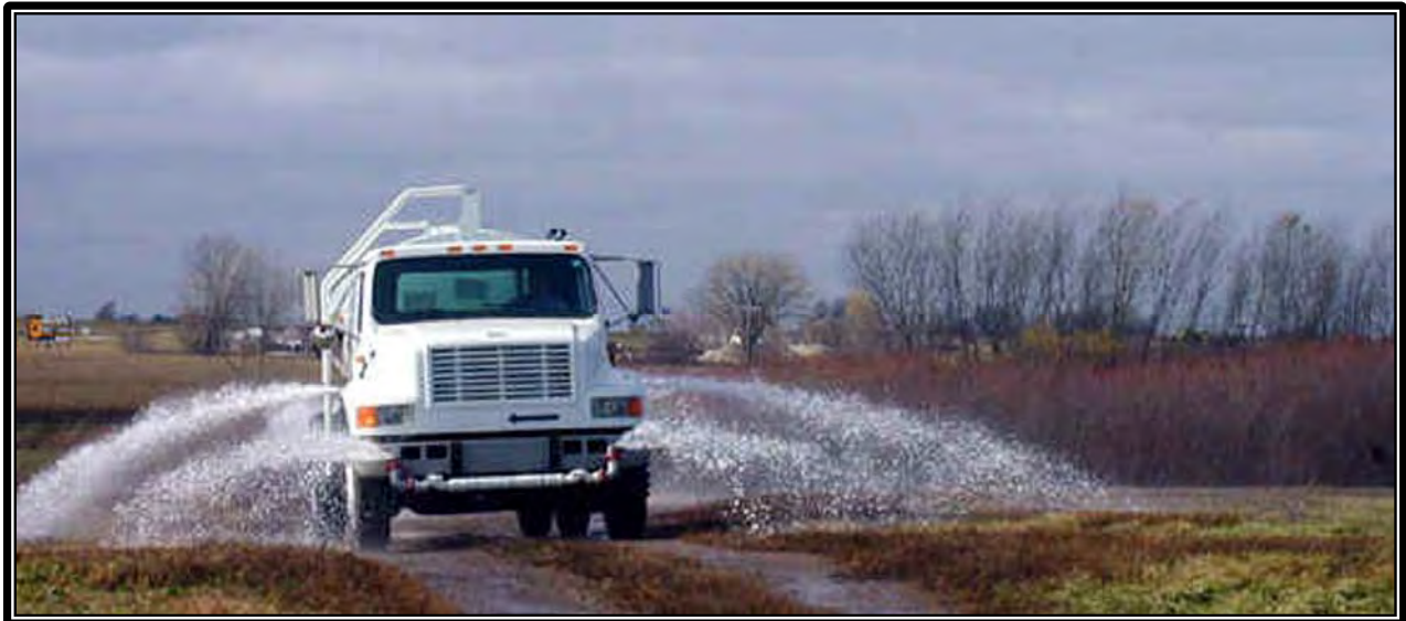
Figure 4.21. Dust Suppression by Water Spray.
