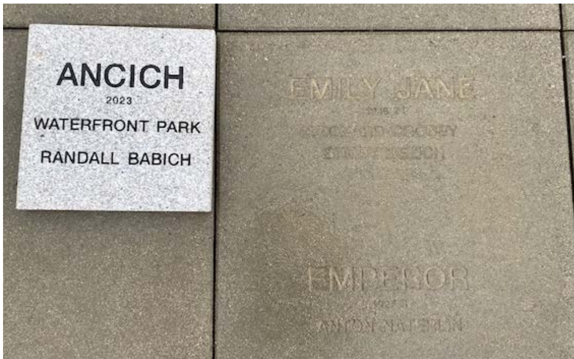
Image 2: Sample Granite Paver Adjacent to Existing Concrete Paver
