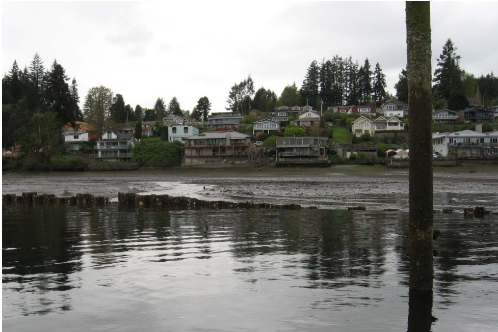
Photo 21 – 2017 (May 1) photo looking northwest at sheetpile wall and main stream channel flowing toward it. (courtesy Parametrix)
