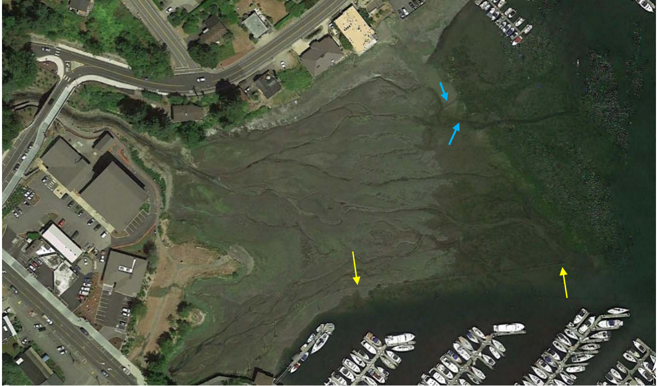
Photo 13 – 2014 aerial photo, after completion of new Donkey Creek outfall channel and bridge, construction of sheetpile wall (yellow arrows; seaward end at right arrow) paralleling marina basin, and re-dredging of marina basin. Mound is crossed only by the same two channels (see blue arrows) as in 2012. One of the main distributaries from Donkey Creek plus the coalesced channel from the Austin Estuary outfall join and flow into the basin between the eastern end of sheetpile wall and pipeline berm. Turbidity plume is visible in water, continuing between two docks at lower right. (Google/USGS, 7/10/2014)
