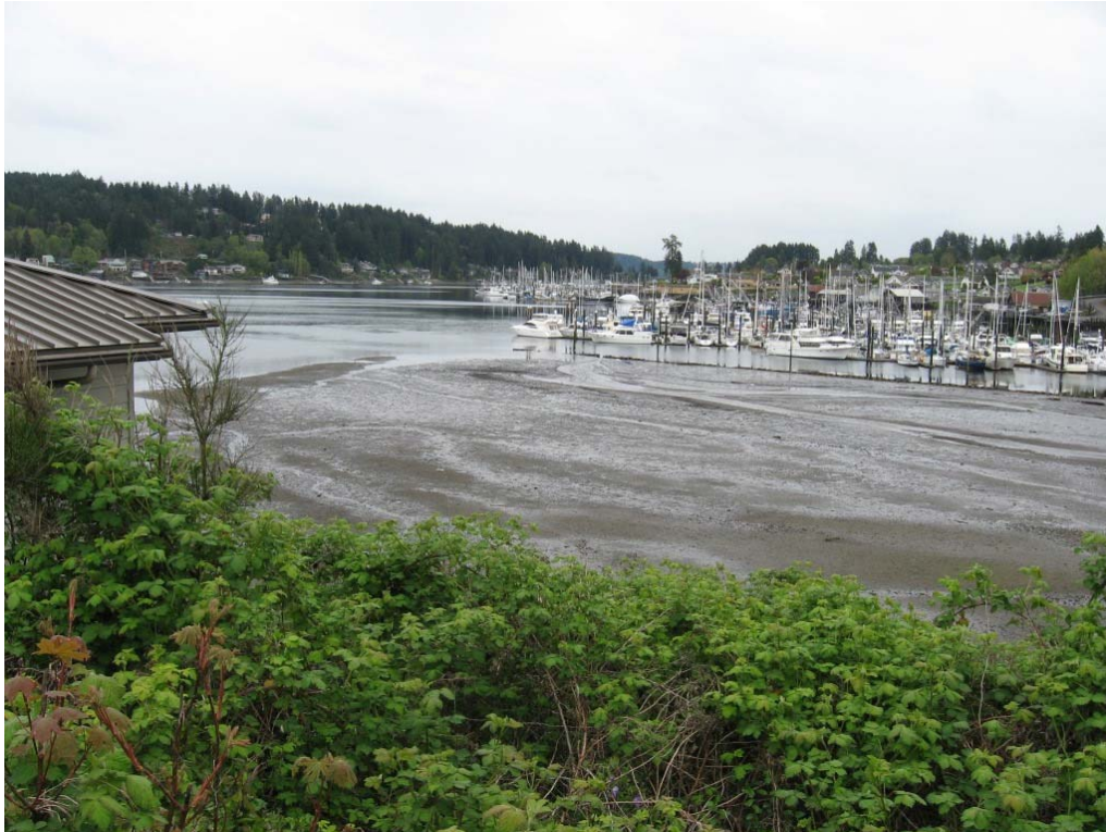
Photo 20 – 2017 (May 1) photo looking east, showing pipeline mound at left and combined main creek channel at center flowing toward sheetpile wall. Mound still largely intact, with channel since 2012 at left (partly obscured by building). (courtesy Parametrix)
