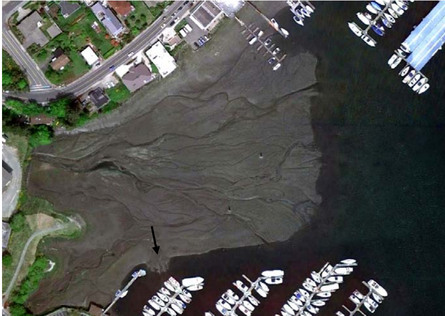
Photo 11 – 2010 aerial photo, just prior to start of WWTP outfall pipeline construction. More Donkey Creek distributary channel changes. Ongoing sediment deposition from channel incursion from Austin Estuary outfall has caused continued fan growth into marina basin (black arrow). (Google/USGS, 5/14/2010).
