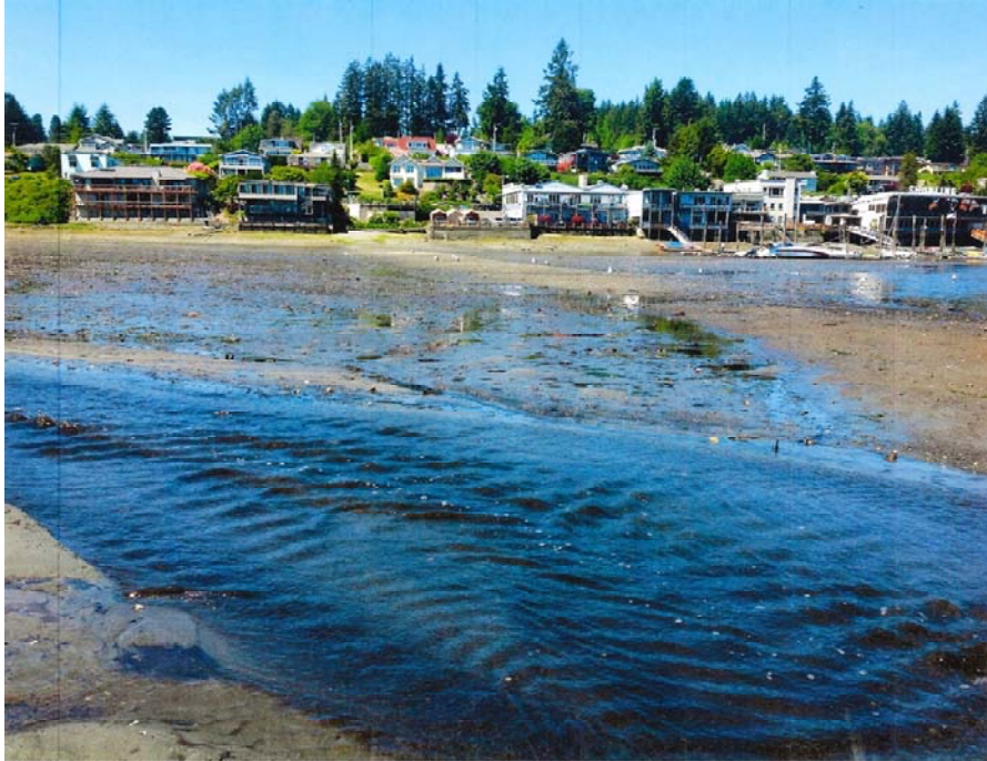
Photo 16 – 2015 (Spring) photo looking northwest. Main combined channel of Donkey Creek and Austin Estuary, diverted by outfall pipeline berm (at right) and flowing to east of sheetpile wall. (photo courtesy of the marina)
