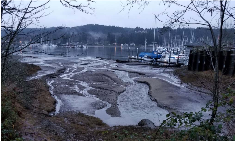
Photo 23 – 2018 (January 24) photo looking northeast. Austin Estuary outfall stream. Murphy's Landing Marina on right, with low sheetpile wall visible to left of high wall. Streamflow was not turbid despite recent abundant rainfall over several days through the day of observation. Stream bottom is eroded to gravel lag, and fresh sand deposition is apparent on top of bars. Likely due to reworking of delta sediment.
