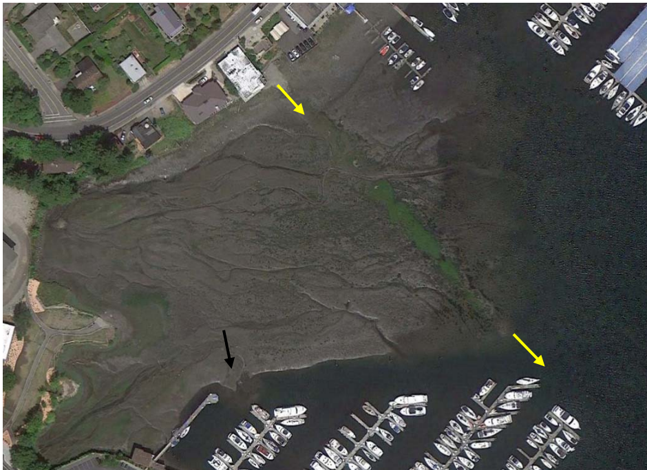
Photo 12 – 2012 aerial photo, after construction of WWTP outfall pipeline (yellow arrows) with backfill mound (arrows show alignment; pipeline is beneath diagonal mound partly seaweed-covered, center right). Mound is crossed by only two channels, at upper center. Other channels that formerly crossed the location of the mound are apparently blocked by the mound. Note that channel incursion and resulting sediment into marina from prior to outfall construction is still present (black arrow). (Google/USGS, 7/12/2012)
