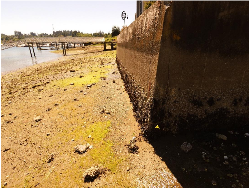
Figure 3. Looking South along baseline / bulkhead from the North
