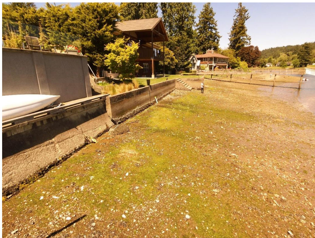
Figure 2. Looking north along the survey baseline / bulkhead from existing dock to the South
