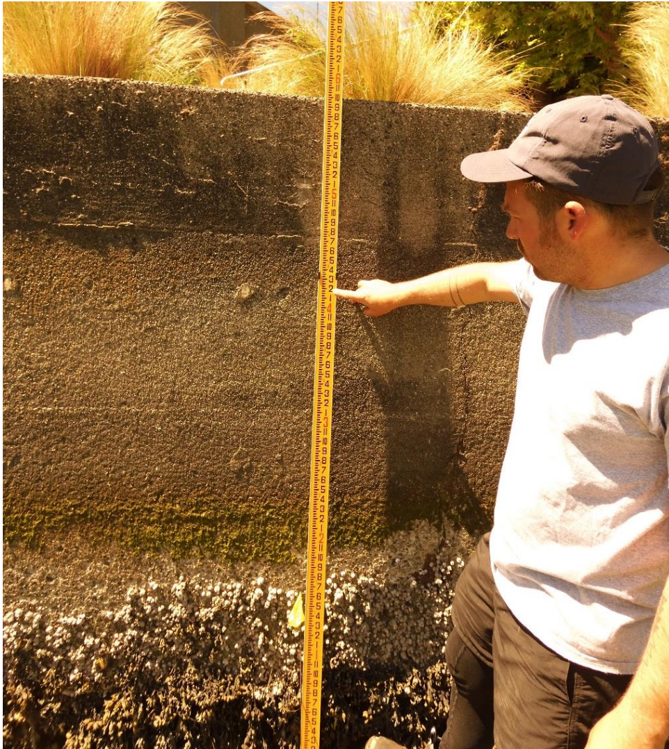
Figure 5. OHWM measured on the bulkhead
