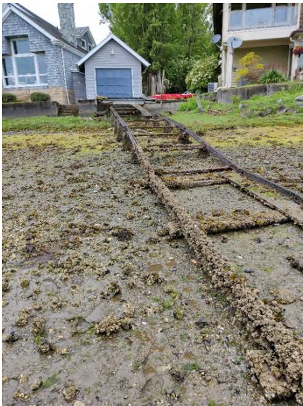
Figure 7. Photos of marine rail and concrete piles to be removed
