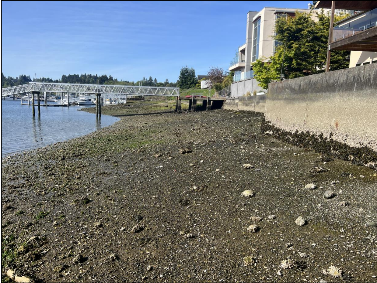
Figure 2 Overview of project towards west
