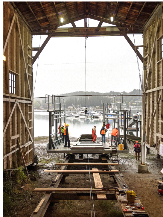
Engineers and volunteers building the inside 'Ways' carriages 2021
