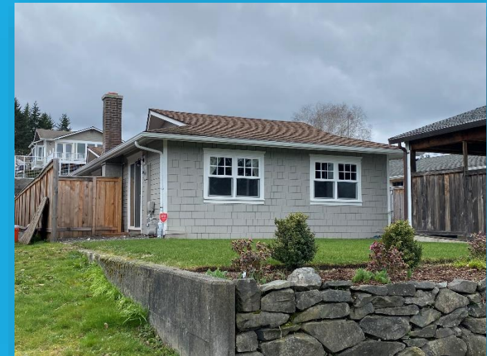
View 3 – Existing front façade
