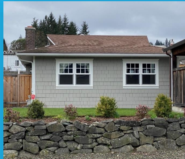
View 2 – Existing front façade
