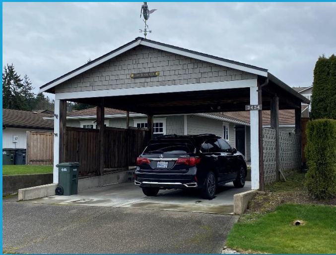
View 1 – Existing front façade
