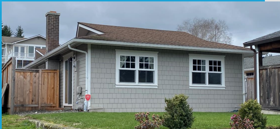
Angled view of existing façade from street
