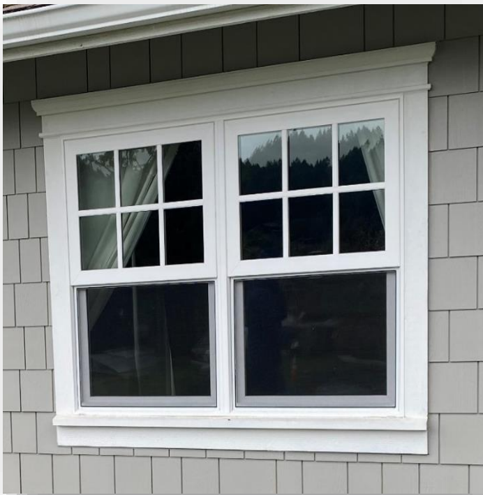
Photos of existing installed windows
