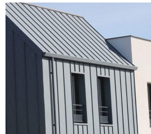
STANDING SEAM METAL ROOF
