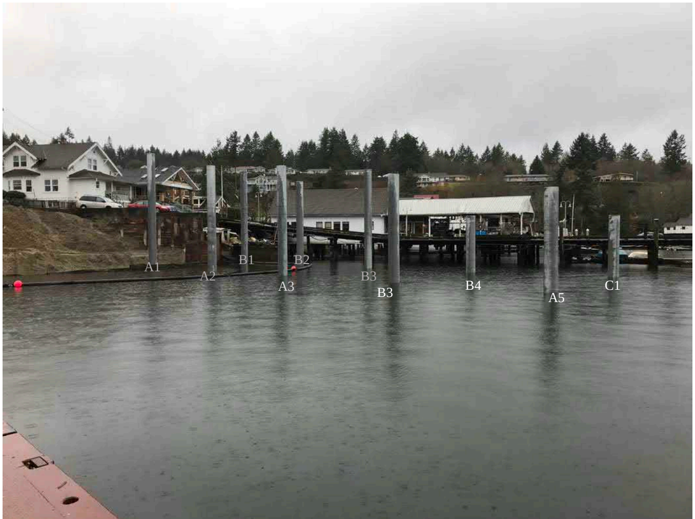
Monitored Piles at Ancich Site (C1,B4, A5, B3).
