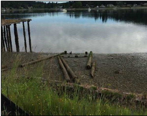
Photograph 7 – Piles in the intertidal
