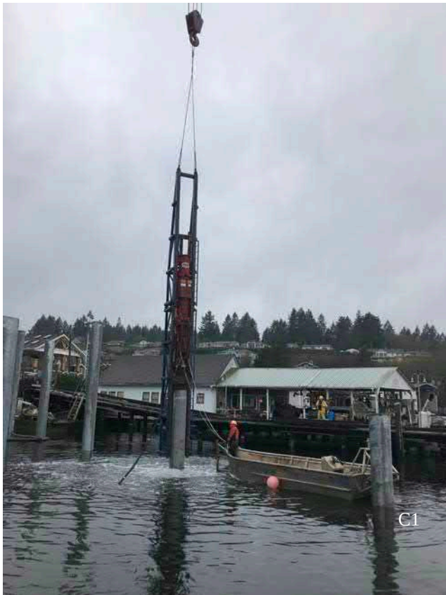
Pile Driving B4 (Bubble curtain ON)
