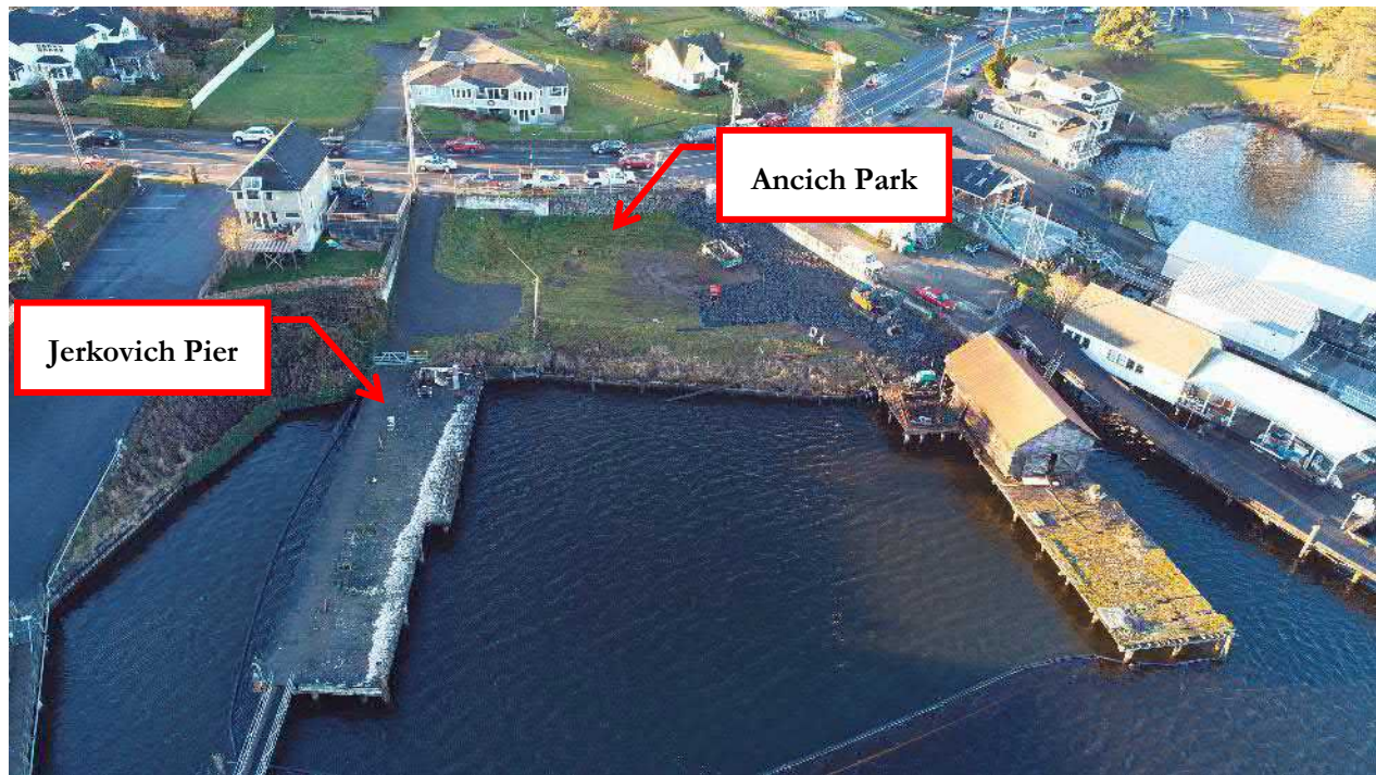
Figure 2. Aerial Image of Ancich Park Mid-Construction
