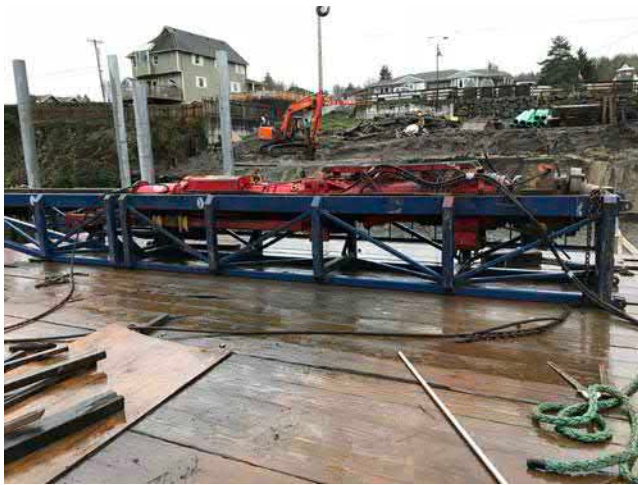
Delmag 32 impact hammer
