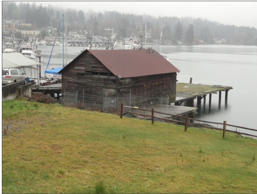
Figure 7-6. Ancich net shed (view northwest).
