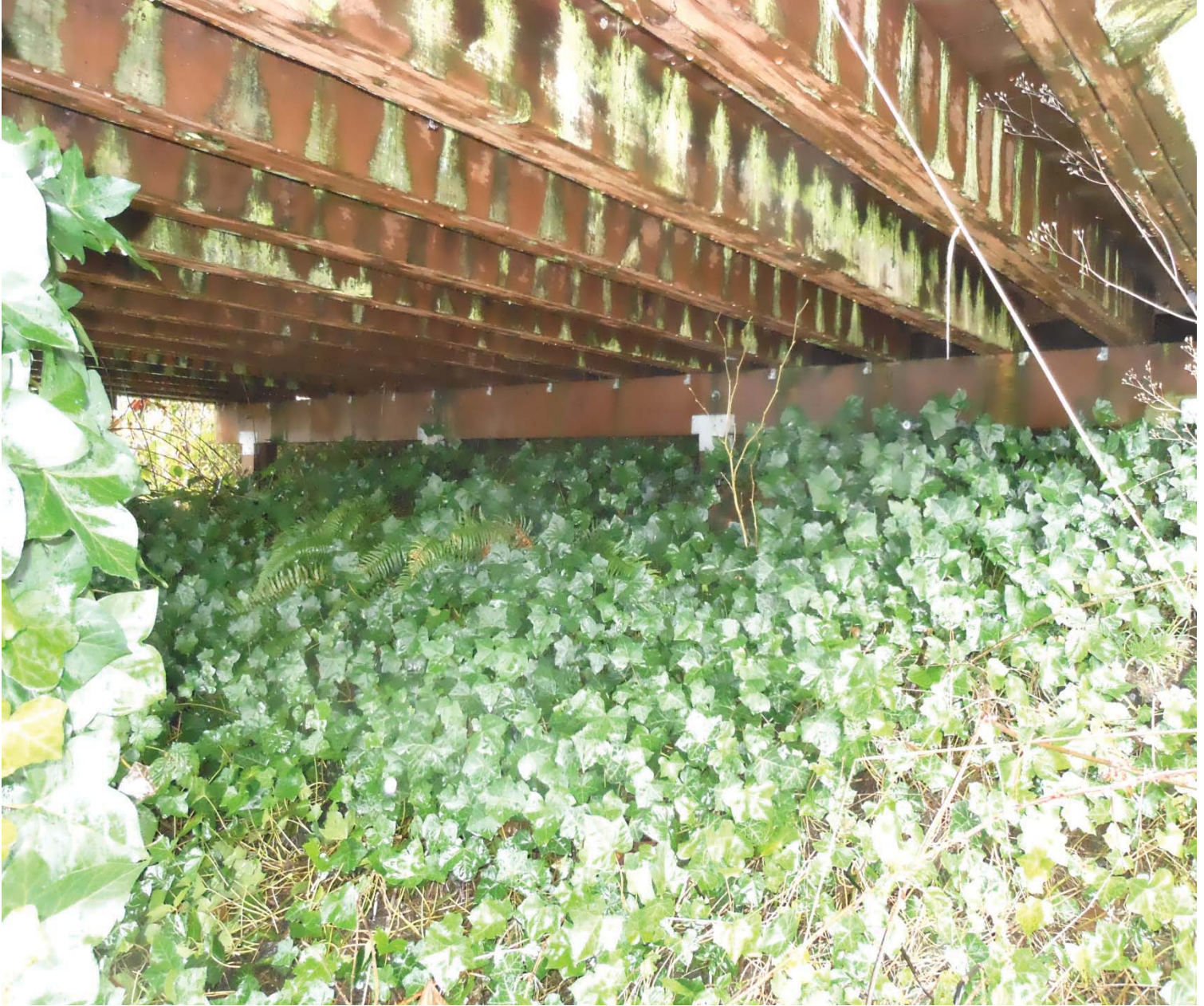
Location of outside heat pump unit as shown on the plans
