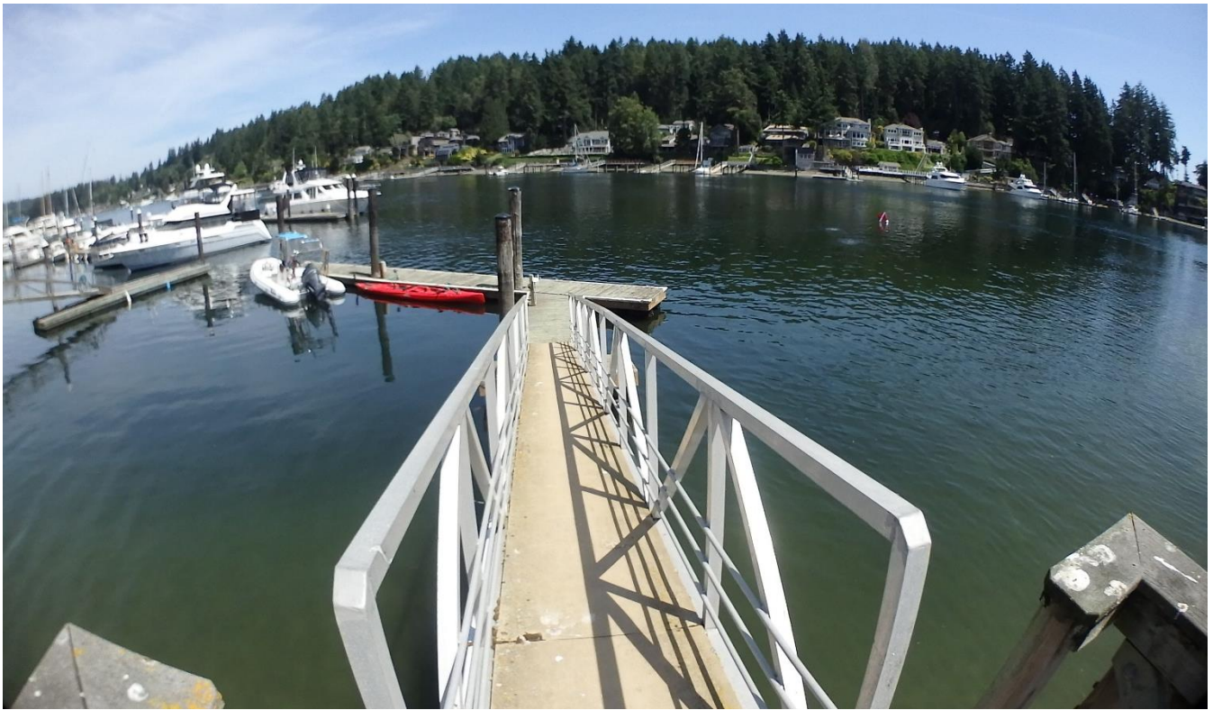
Chatman dock to be removed
