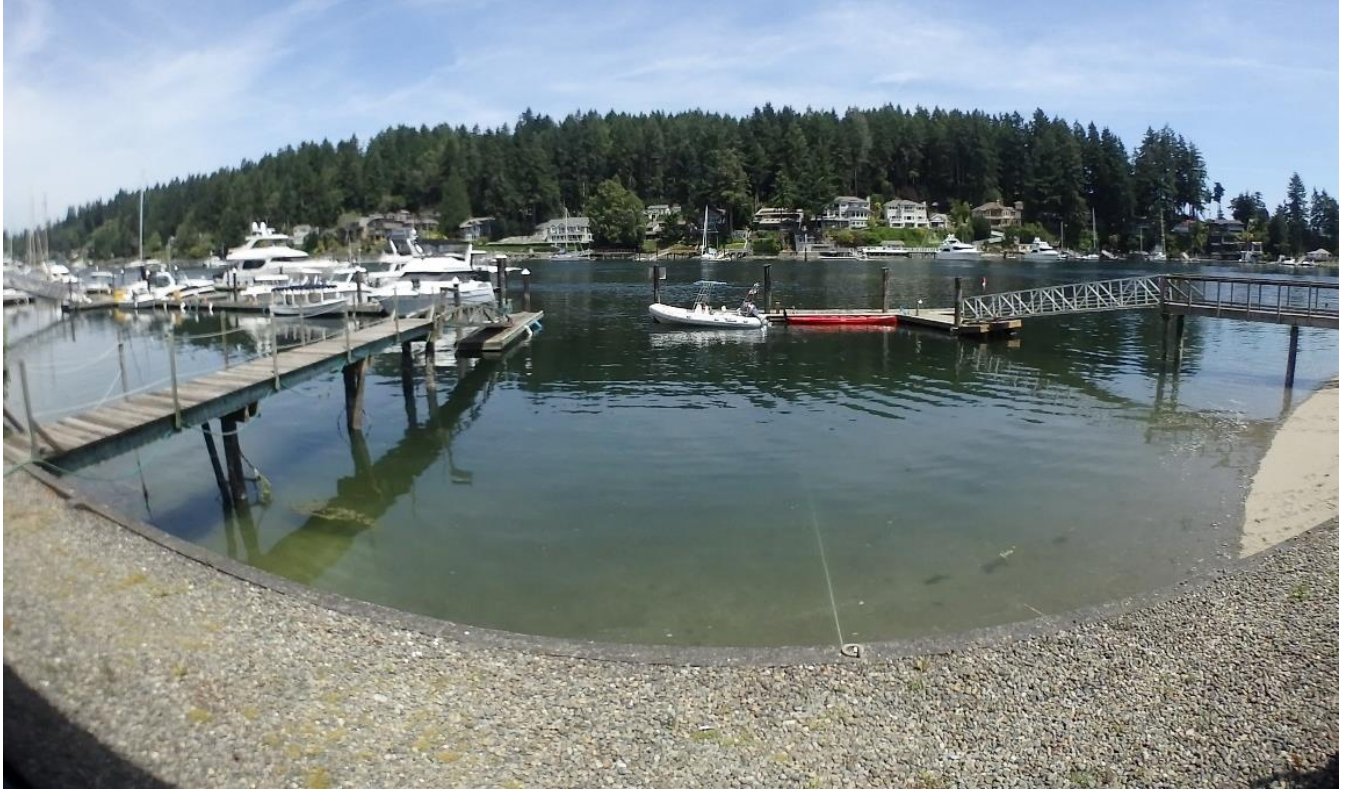
Both docks to be removed-Hodge on the left, Chatman on the right
