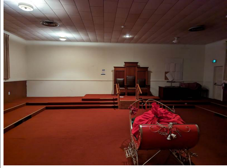
Photograph No. 18 Interior, main floor, looking west Notes: Typical interior condition
