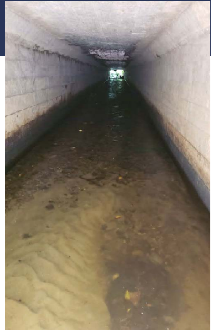
6' X 6' X 146' box culvert (constructed 1970) cataloged as 67% fish barrier by WDFW
