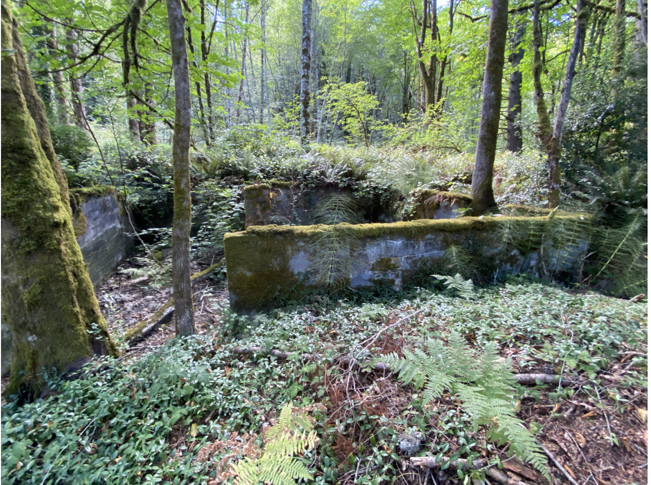
House Foundation in dry season, August 2025
