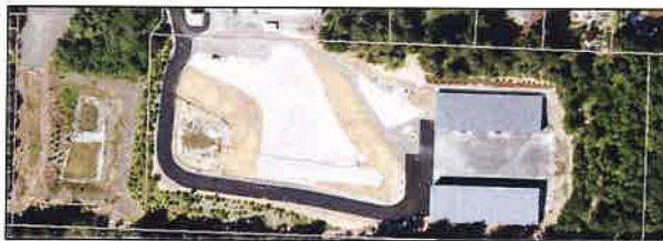
Aerial of Current development
