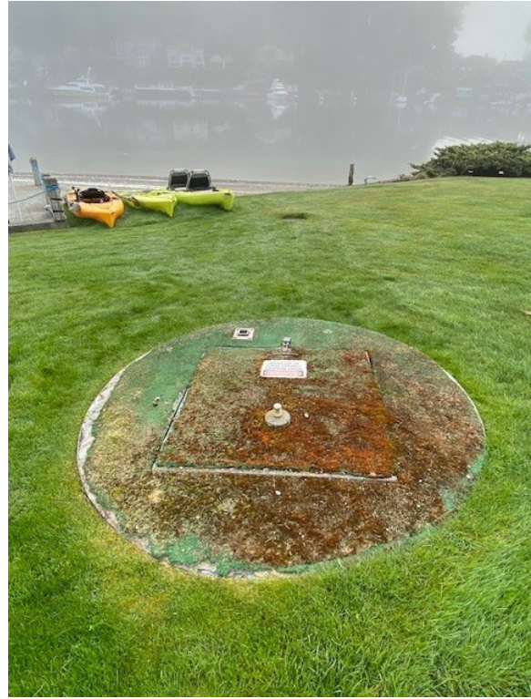
Photograph 2. Lift Station #5 Looking East
