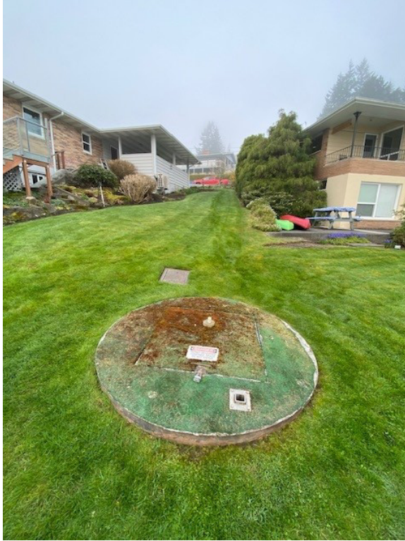
Photograph 1. Lift Station #5 Looking West
