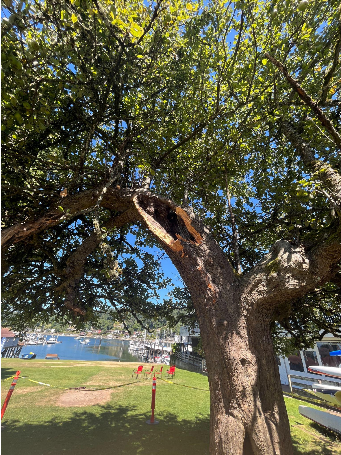
Image B2. The recent large limb failure revealed extensive internal decay that goes from the base of the tree up through the major scaffold branches. There is only a few inches, at most, of holding wood.
