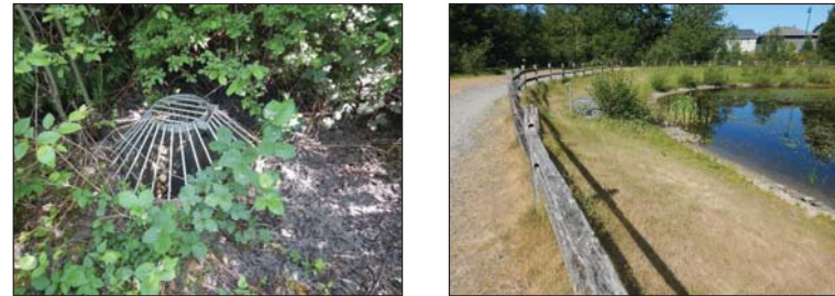
Figure 3. Stormwater Pond Culverts
