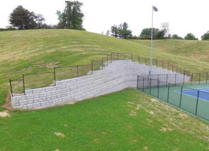
Retaining Wall - With Fencing
