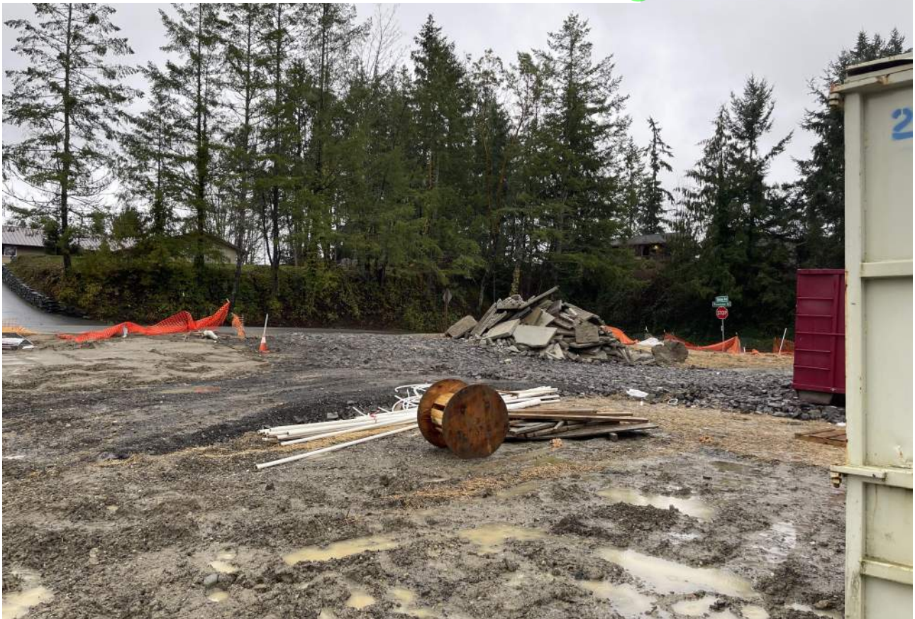
VIEW LOOKING SOUTH-EAST STANDING ON PARCEL E
