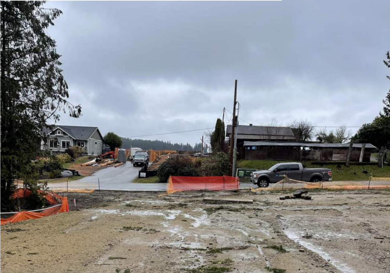
VIEW LOOKING EAST STANDING ON LOT 02
