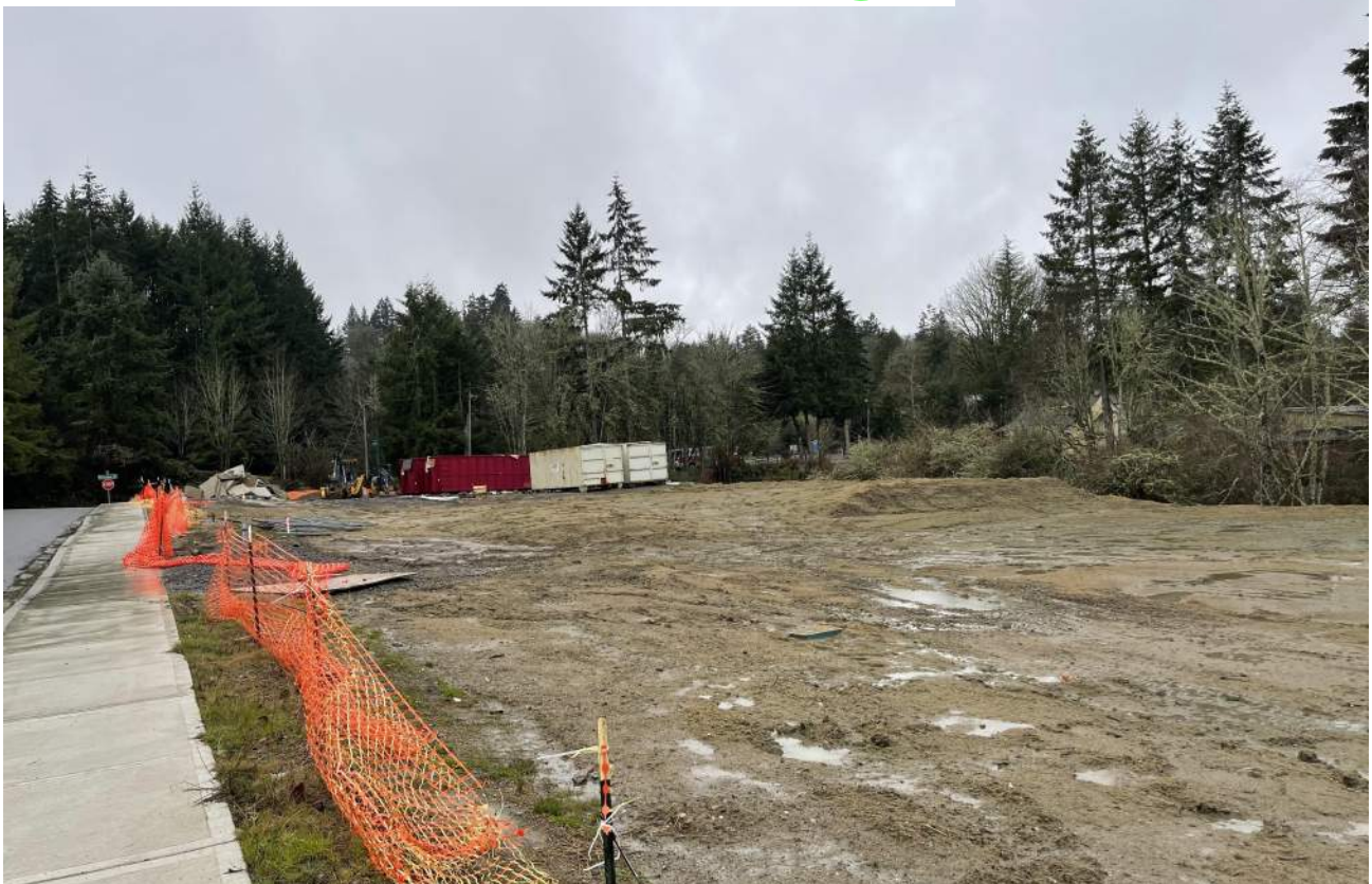
VIEW LOOKING SOUTH STANDING ON PARCEL B
