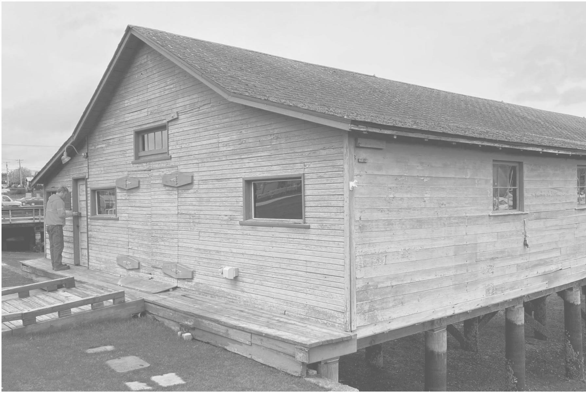
5G CLOSE UP VIEW OF SOUTHEAST CORNER OF BUILDING SCALE: N.T.S. Image 1
